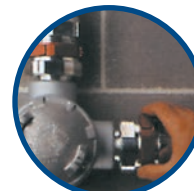
6. Insert cable and tighten red union
