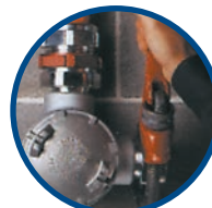
5. Install hub on enclosure
