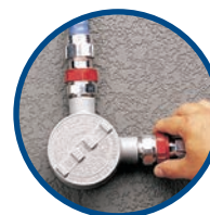
7. Insert cable and tighten red union
