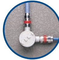
6. Insert hub on enclosure
